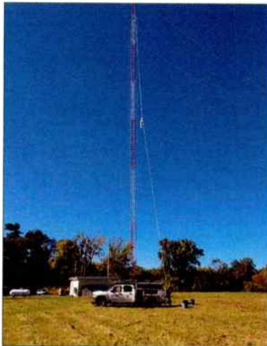
Hoisting the WISP Antennas
