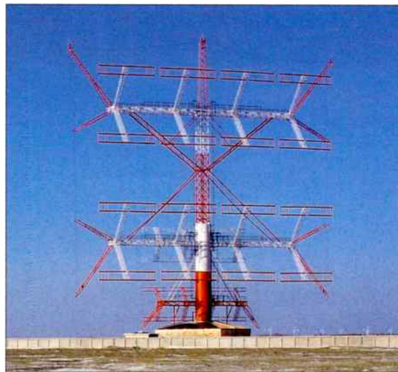
Ampegon Antenna Systems Curtain Antenna
