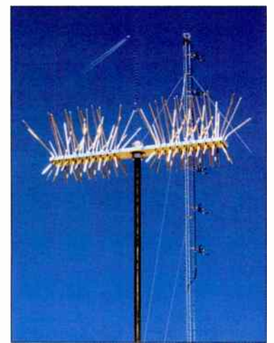
The GS-3: Different adaptations of multiple point dissipaters.
