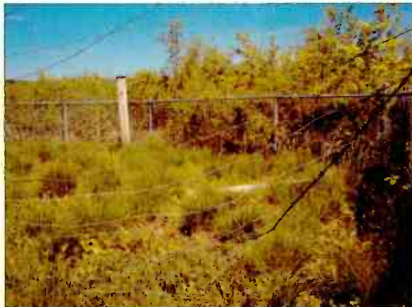
Suspended ground system as it should not be.
