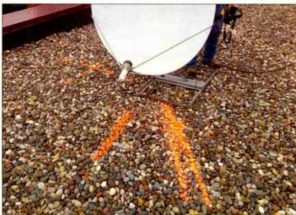
The orange lines are the look angles to the three satellites MPR needed to see. The KU dish is the receive antenna MPR used to verify that we could see all three satellites.
