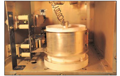
New Plate Blocker Installed
