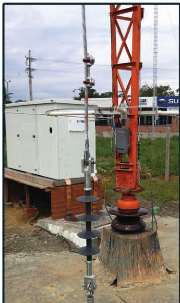
MODEL KSA-VCTB-10 KINSTAR LOW PROFILE ANTENNA ON THE AIR IN COLOMBIA, SOUTH AMERICA
