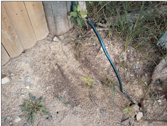
New Fence Post = Cut Sample Line
