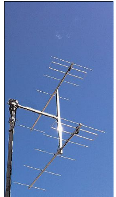
Figure 2 – Beams on Tower
