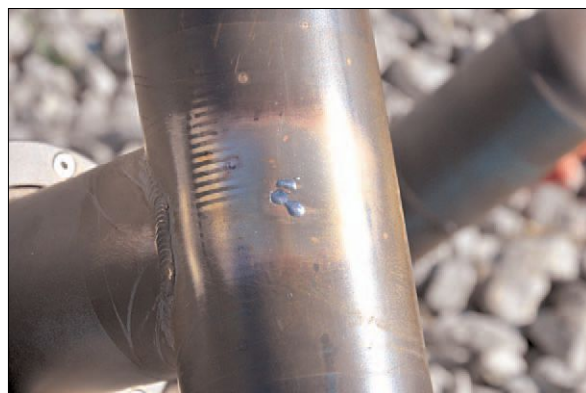
Solder fills the hole.
