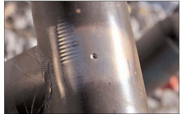
Burrs removed and prepared for patch.
