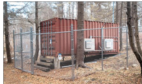
The WNSH transmitter shelter.
