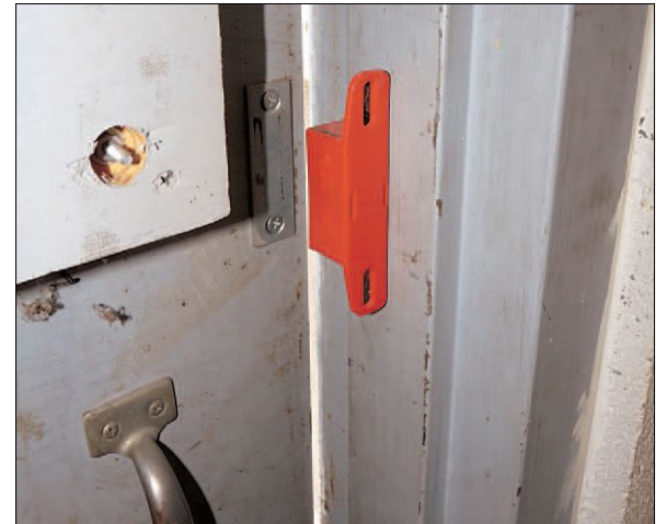
A magnet keeps the door from swinging open.
