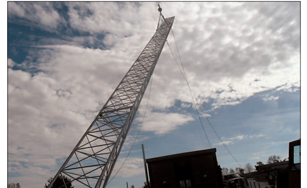
New tower and DA installation in McKee, KY.
