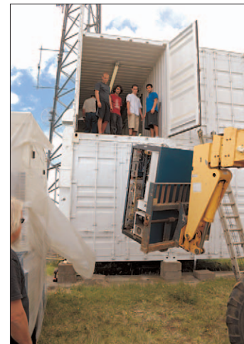
The Nautel NV20 gets moved into its new home.
