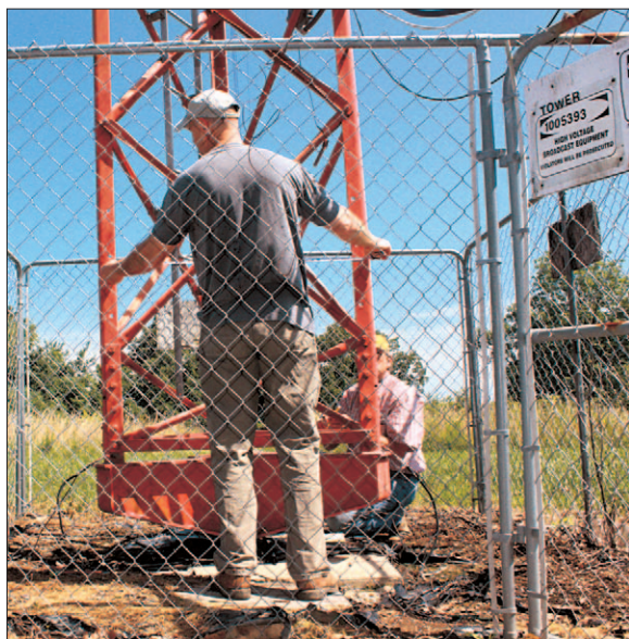
Max Brown of Broadcast Connection and Ernie Jones P.E., of CEI Engineering, measure a tower for a structural analysis.
