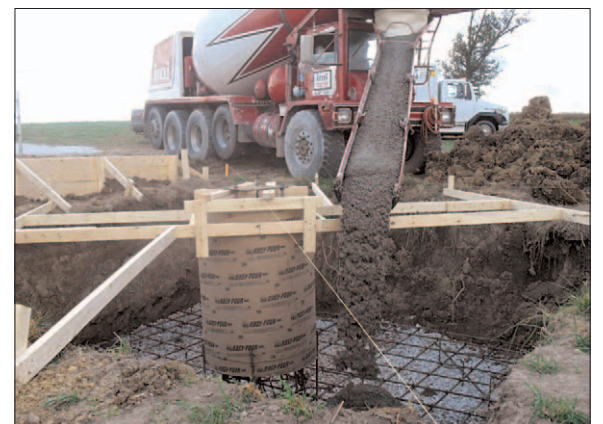
New tower foundation Greencastle, IN.
