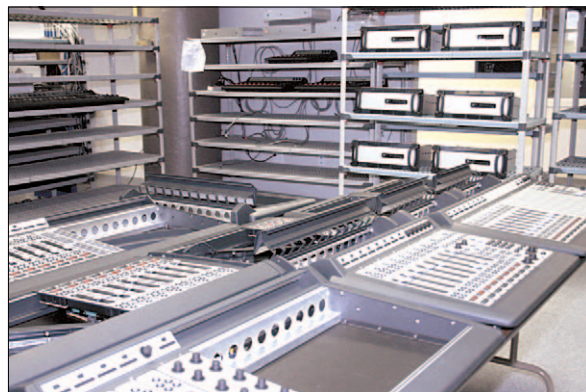
Axia Consoles tested and ready for burn-in.
