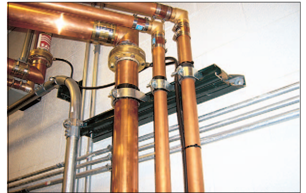
Hard line mounted with a resilient rigid mount.
