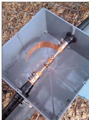
A look at the splices of the emergency cable.
