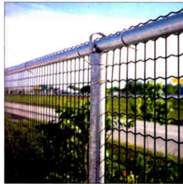
This nine gauge fence provides more security.
