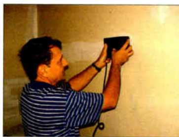
John demonstrates how to locate a hidden conduit box with a tape eraser.
