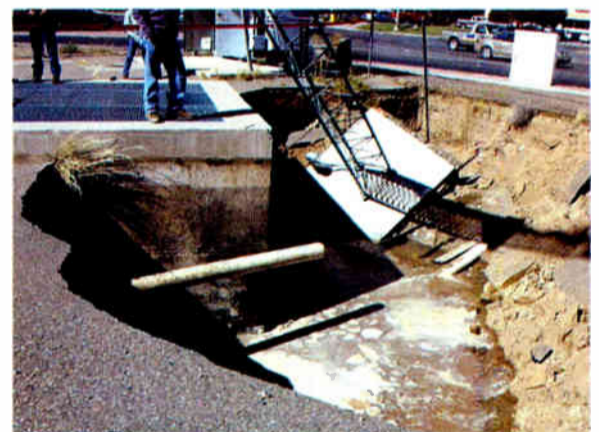
Our thanks to Rico Gonzales of Advanced Tower Services for the pictures.
