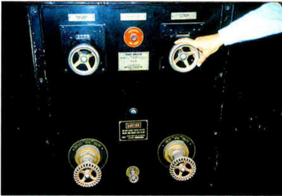
The EMERGENCY SHUT DOWN button is top center.
