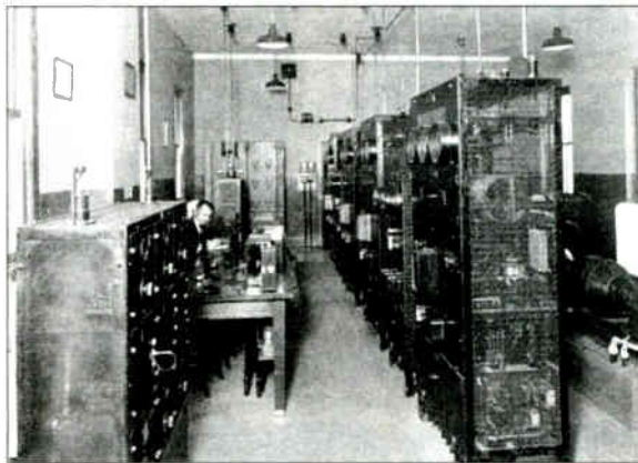
RCA Transmitter House in NY, with four GE transmitters installed in a row to feed the RCA stations.
