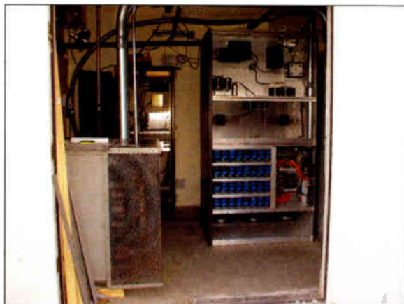
After installation – a comfortably tight fit.
