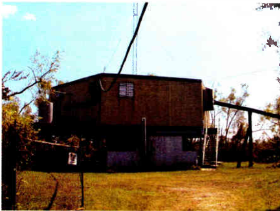
WWL's transmitter site was built elevated and was undamaged, but difficult to access.
