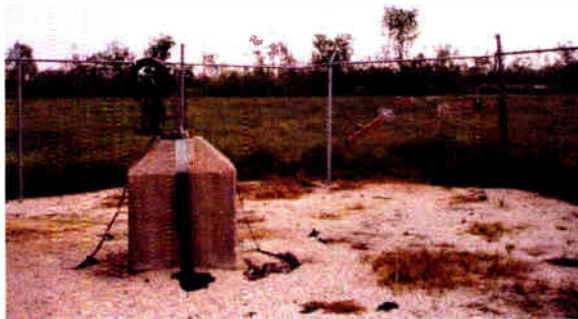
Where has the WYLD tower gone?
