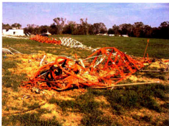
Katrina smacked the WUSW/WNSL tower right down to the ground.
