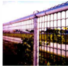
This nine gauge fence provides more security.
