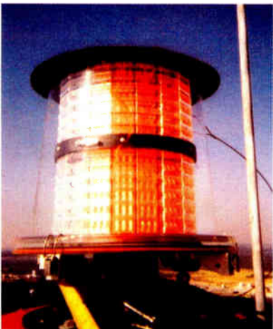
LED beacon re-installed at the 499' (top) level.
