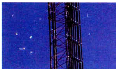
Falling ice can be worse than loose bolts.
