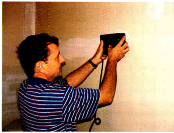
John demonstrates how to locate a hidden conduit box with a tape eraser.
