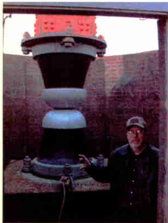
Watt Hairston, CE of WSM stands next to the base insulator.
