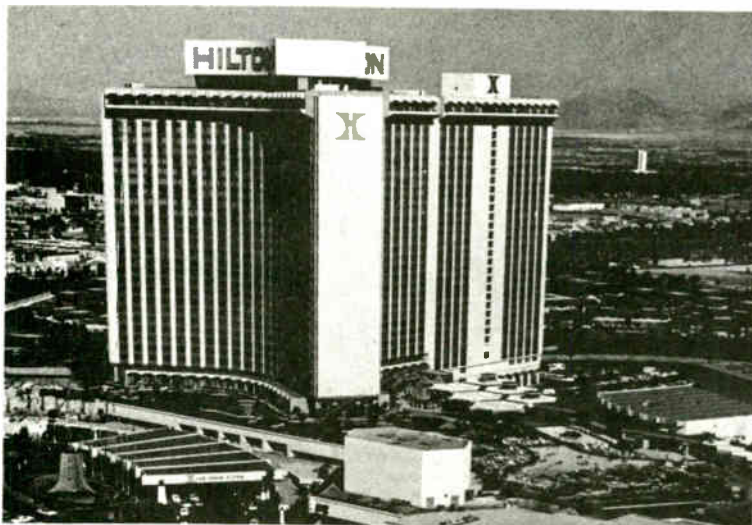
LAS VEGAS HILTON TOWER BEHIND CONVENTION ENTRANCE
