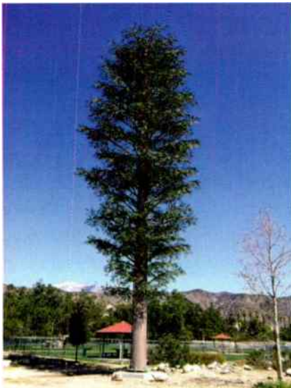
A Chameleon Engineering simulated view of a eucalyptus tree with 8-foot branches for a camouflaged antenna site.
