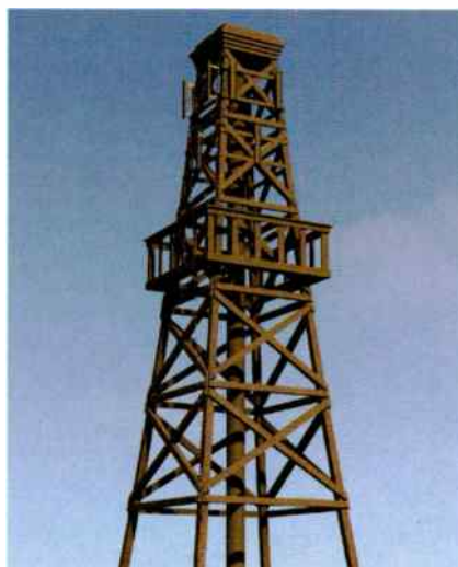
A Chameleon Engineering 3-D simulated model of a proposed antenna site disguised to look like an oil derrick.
