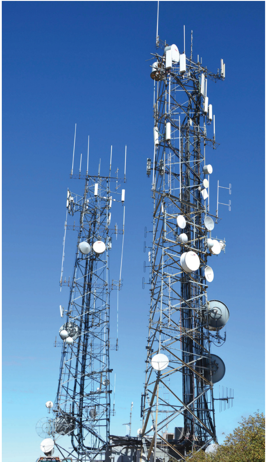
Making a site visit to inventory what is on the tower can easily be expensive, especially if the tower is on a mountaintop or at a remote location. The cost of having the survey done by a local surveyor located near the tower can be considerably less than having it done by a worker who travels from a faraway location. The accuracy can be easily documented because of the files produced by the laser survey.
