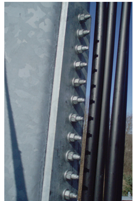
Photo 7. Bolted MP2 flat plate using Ajax bolts.
