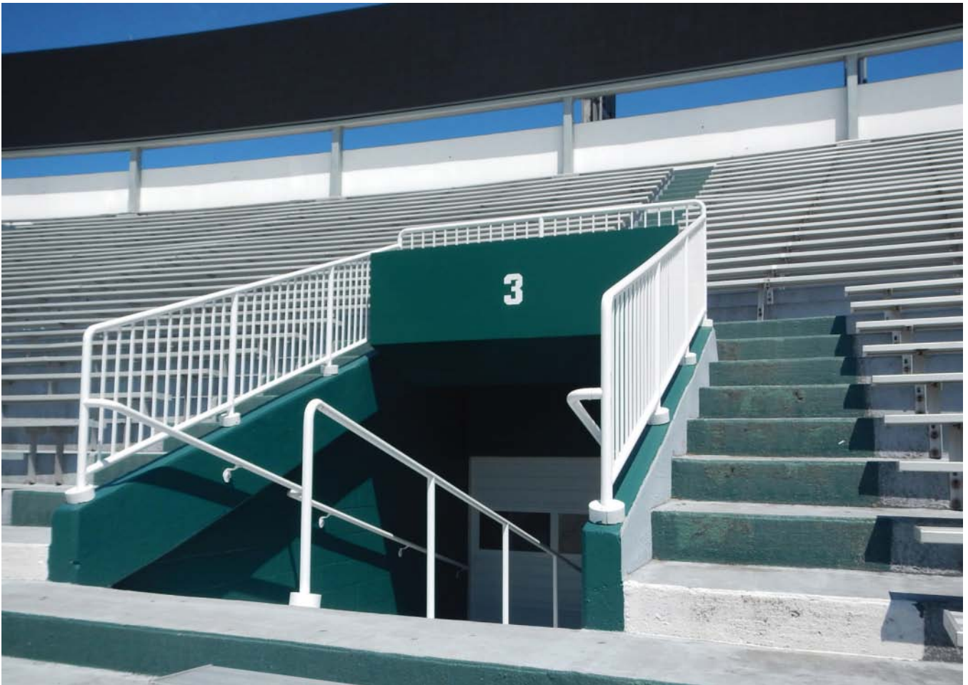
Hiding distributed antenna system antennas, a panel bearing the digit 3 and made by Stealth Concealment Solutions of North Charleston, South Carolina, delivers signals to serve sports fans who come to Spartan Stadium in East Lansing, Michigan.
