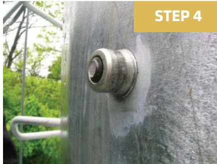
Photos 3–6. These photos show step-by-step how to install the Huck lock-bolt fastener.
