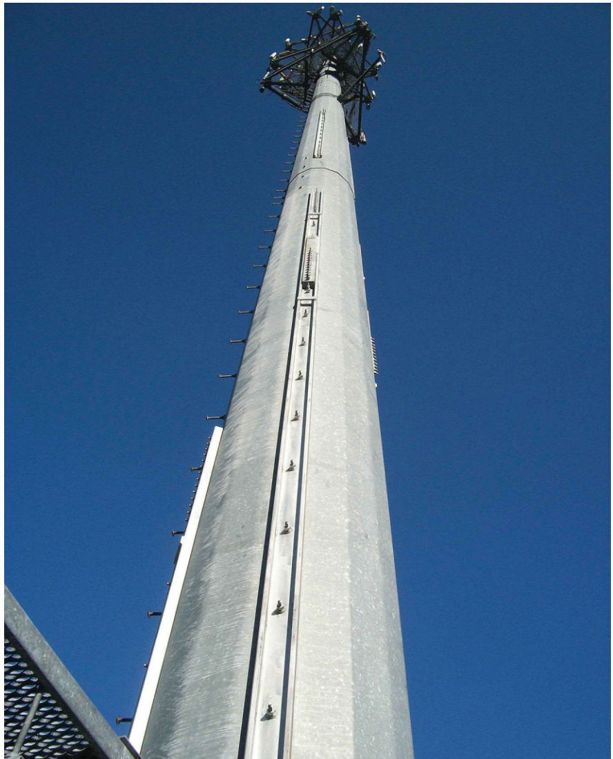
Photo 2. A bolted MP3 channel.
