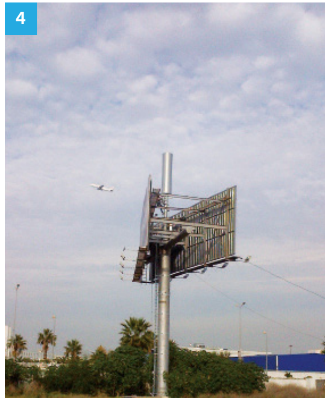
A sequence of images shows the installation of a macrocell canister on a monopole that supports a billboard, disguising the cell site as an advertising structure. Photos courtesy of CommScope
