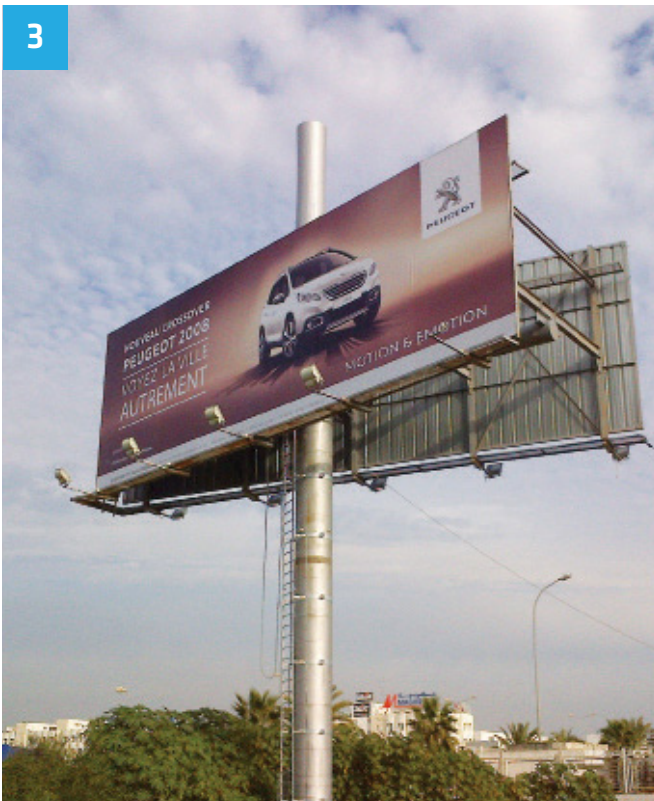
A sequence of images shows the installation of a macrocell canister on a monopole that supports a billboard, disguising the cell site as an advertising structure. Photos courtesy of CommScope
