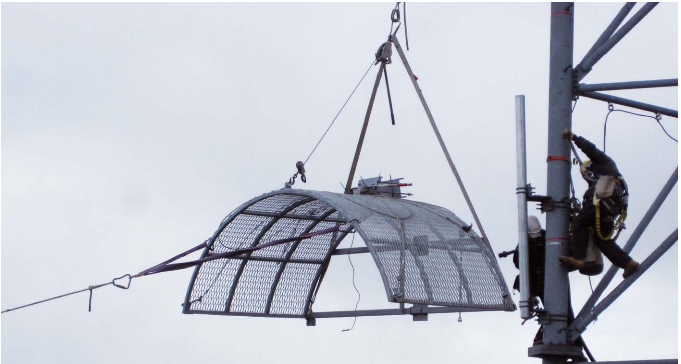
Ice shield installation on Mt. Kearsarge.
