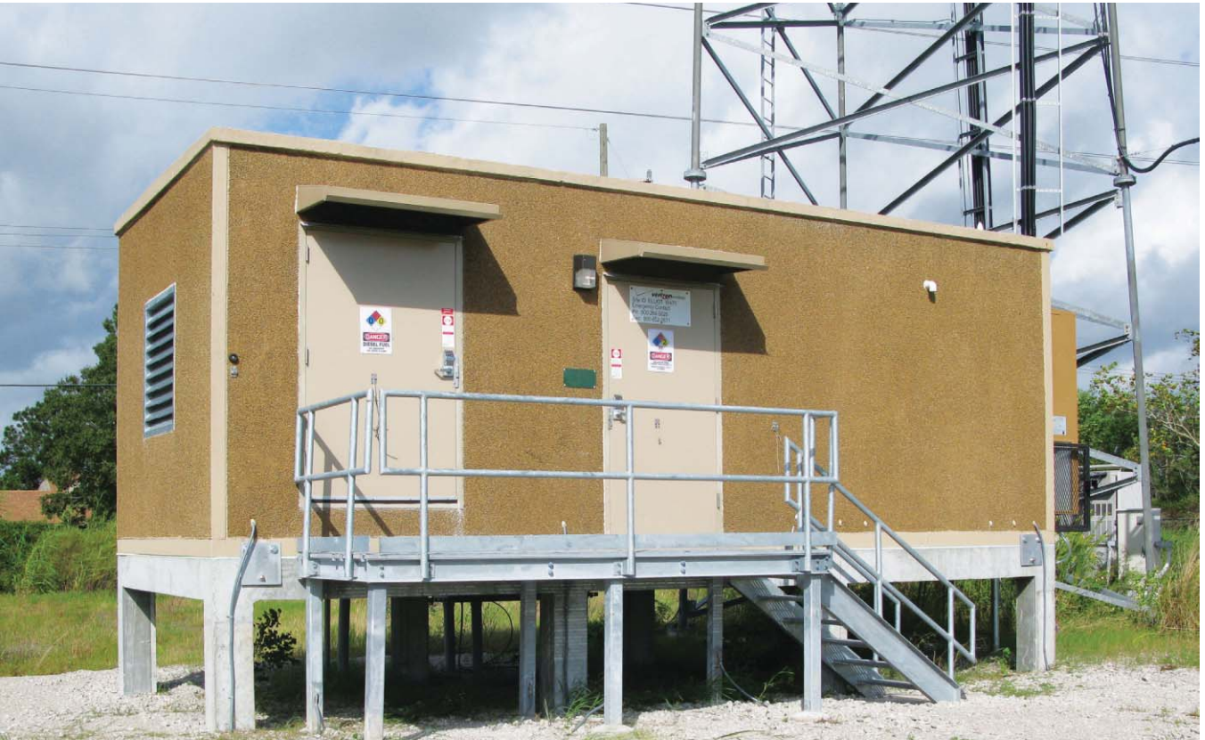
Crews installed the chain wall for the East Baton Rouge Sheriff's Office 911 system in a single day.
