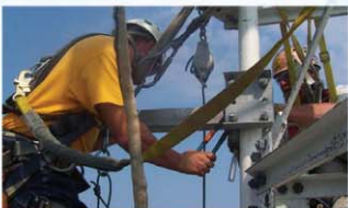
Tower and Antenna Maintenance
