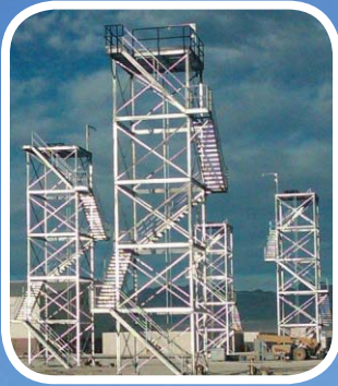
Crech Specialty Structure
