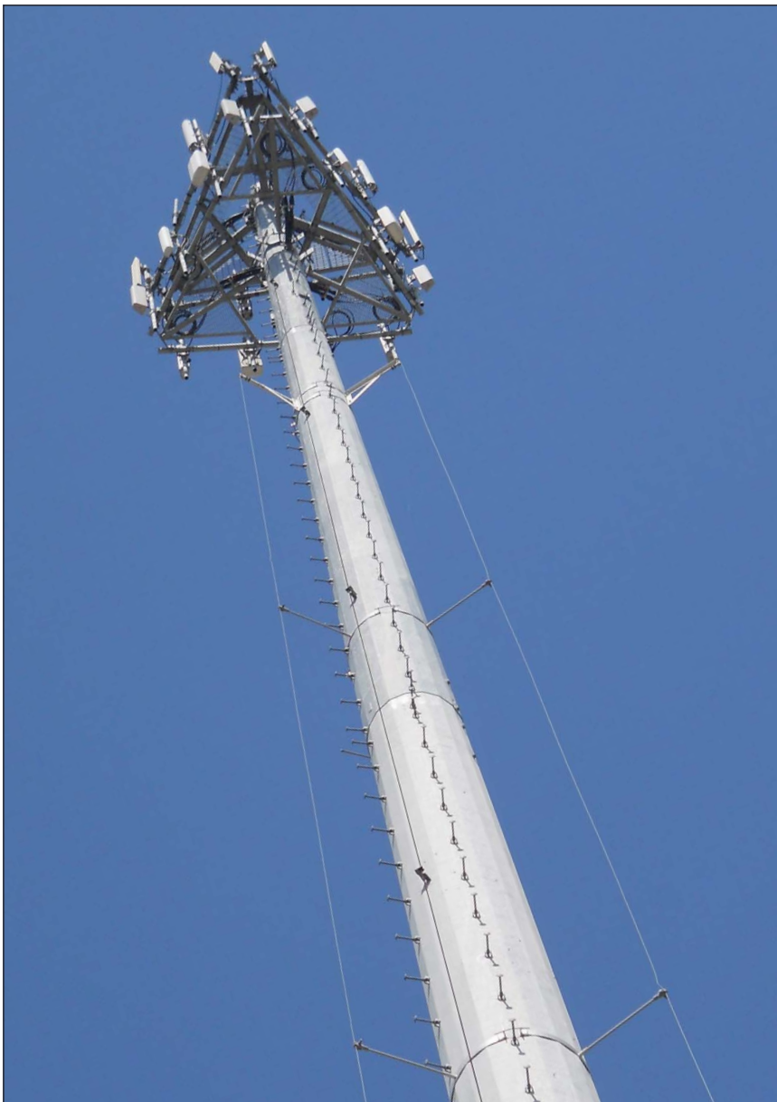
Wires that parallel the tower form a skirt as part of a system to detune the tower, which means to modify its electrical wavelength so it does not reradiate the AM station signal. Photo courtesy of Waterford Consultants/Larry Giessman
