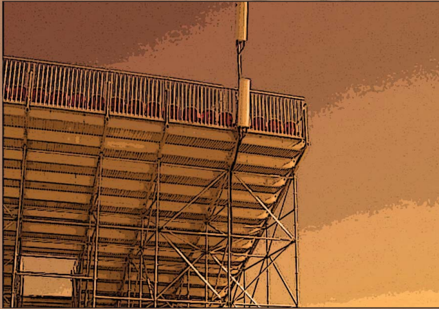
Photo 7. While the amphitheater was under construction, some antennas were placed on nearby grandstands to deliver a signal into the amphitheater. Photo courtesy of ExteNet Systems.
