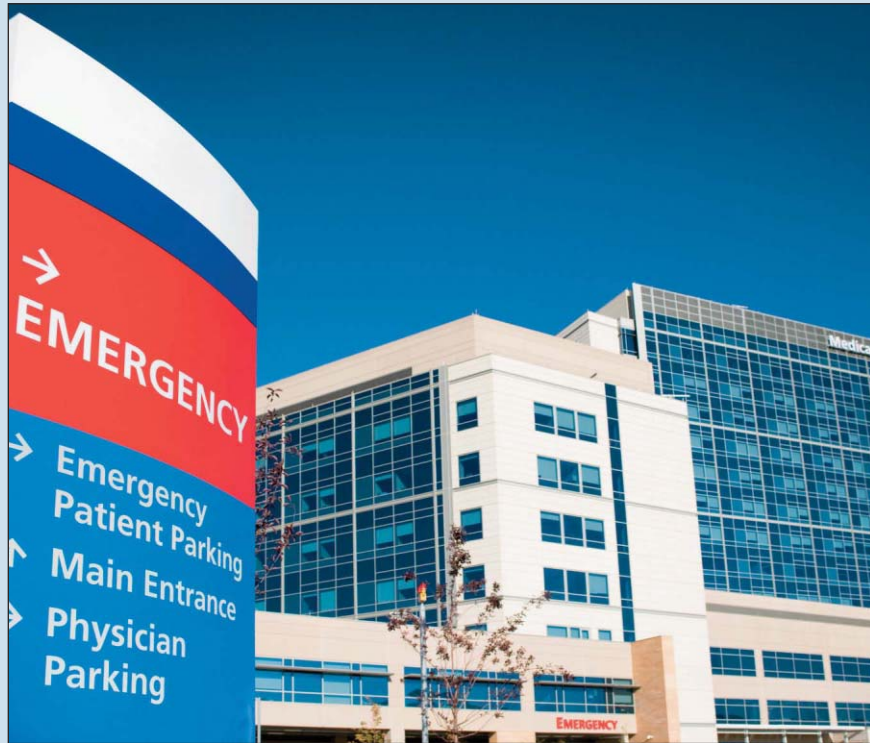
Hospitals that provide open DAS platforms give visitors the ability to stay productive with reliable cell communication. DAS also improves internal staff communication and electronic asset tracking.
