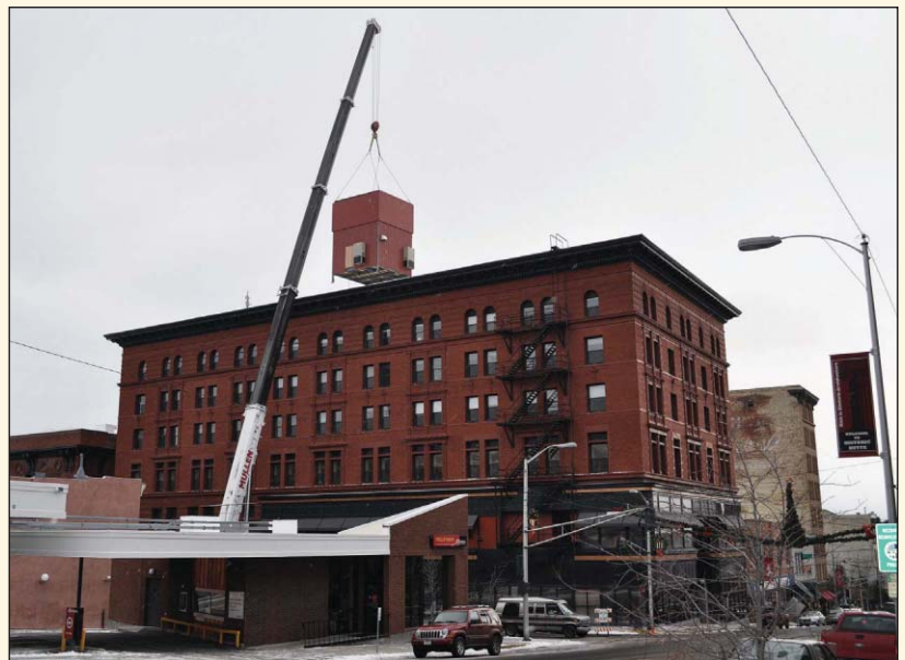
New cell site installation in Butte, Mont.
