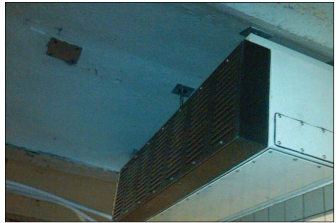
Sealed enclosures protect remote fiber nodes from metallic dust ingress and thus require passive cooling — no ventilator fans.
