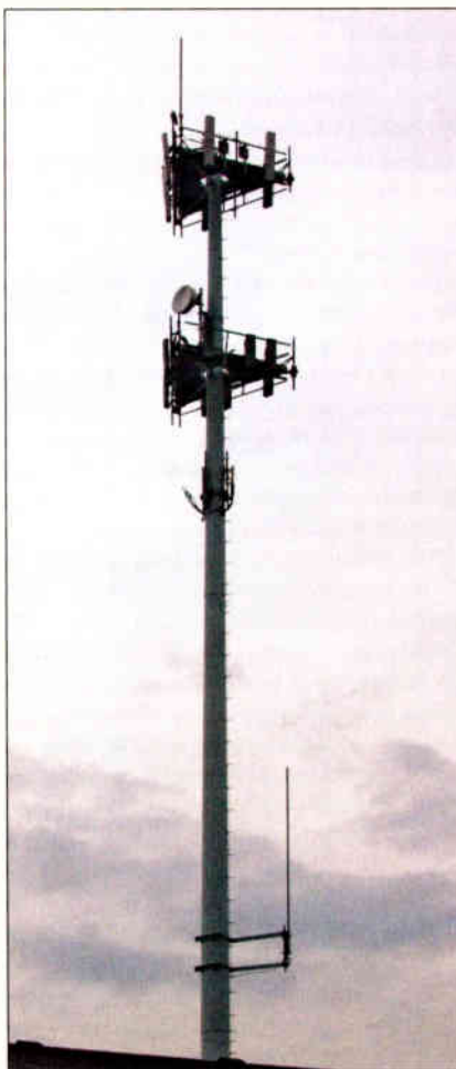
A cell tower sports a side-mounted radio communications antenna that might interact with the monopole, possibly affecting the antenna's RF coverage pattern adversely.
