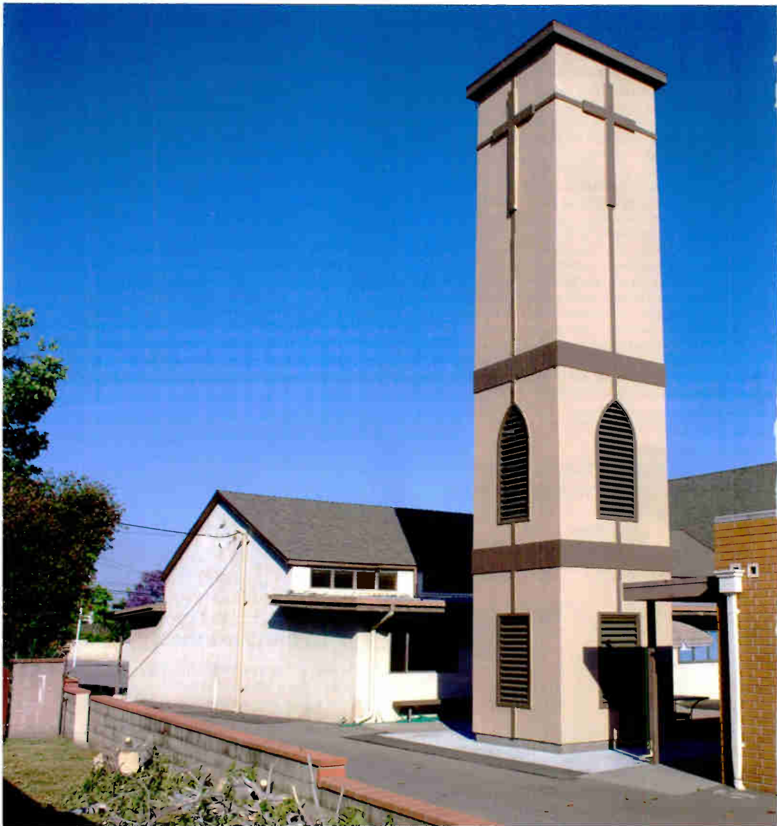
Palisades United Methodist Church, San Clemente, Calif., in recent weeks signed a lease for a monument-style free-standing tower, similar to the one pictured, which will cover a 12-foot by 14-foot area. The 30-year, $1,800-a-month lease was negotiated over the span of two and a half months.
