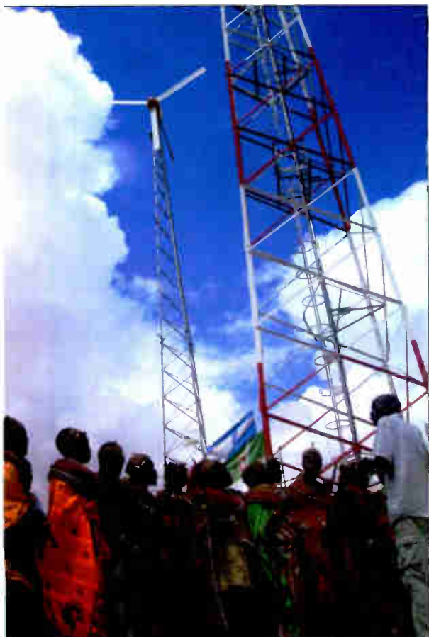
Above: An Air Industrial wind turbine side-mounted on a wireless telecommunication tower near Beech Mountain, N.C., delivers as much as 400 watts with a 30 m.p.h. wind. Such turbines often are connected to batteries to store power and may be combined with solar panels because periods of greater sunlight often have little wind and vice versa. Photos: Southwest Windpower.
