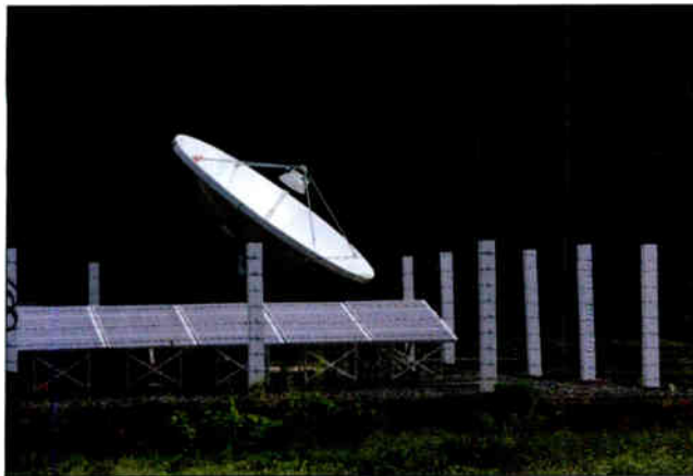
Although solar power carries a pricetag and comes with a footprint that often puts it outside the cost limits of U.S. cell sites, sites in remote locations with no electrical grid service and no fuel availability sometimes use it. Cambodian mobile operator Star-Cell uses solar power at the site pictured above, along with an energy-optimized main-remote base station that consumes up to 50 percent less energy than standard base stations. Photos: Ericsson.
