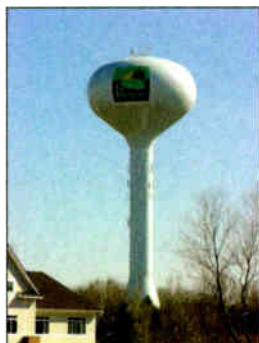
A tank in Vadnais Heights, MN, offers an example of the pedestal type of water tank tower. The nickname for this type of water tank is the 'golf ball and tee.'
