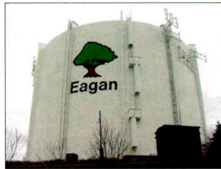
Tanks placed on high ground may need no elevation above the grade to sustain water pressure, and when their walls are high enough, they still offer favored antenna mounting space.
