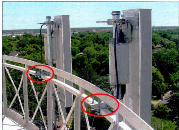
Increased use of beam clamps can reduce or eliminate damage to water tank exterior or interior surfaces or both. Left: A beam clamp secures a coaxial cable. Right: Another type of clamp designed for attachment to structural angles is part of a mounting assembly for two panel-style antennas.
