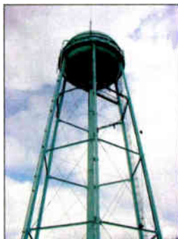
An elevated or legged type tank is supported by steel columns placed around its perimeter. Though inexpensive to construct, today it represents the least popular design.
