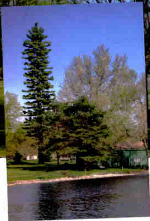
Two views of the monopine concealment pole at the Leawood South Country Club golf course in Leawood, KS. The pre-existing, green-painted maintenance shelter near the base of the pole was lengthened to house base transmitter station equipment. Antenna feedlines between the shelter and the pole are buried. Eight newly planted pine trees circle the pole and are intended to further conceal the site as they grow. Sabre Towers & Poles fabricated the pole.
