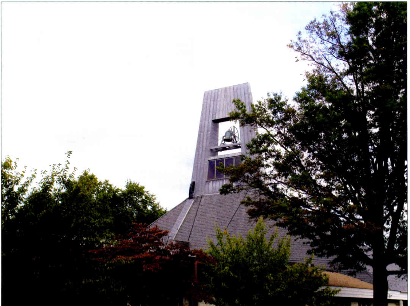
Even a modern bell tower can lend itself to a concealed telecom solution. Photo: John Baptista, CMX Engineering.
