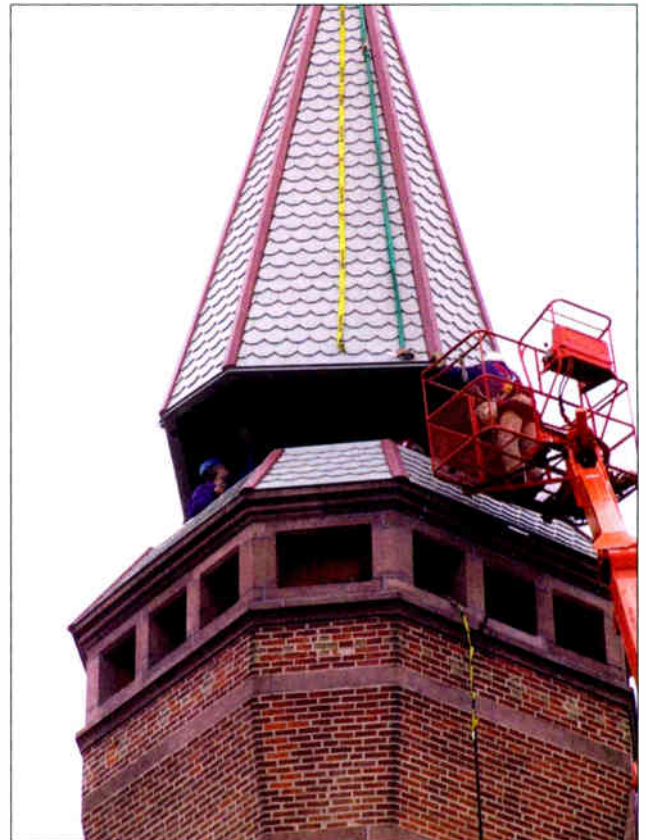
Typical steeple installations utilize readily available manpower and equipment. Photos: Fiberglass Specialties.
