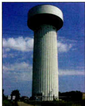
A fluted steel column supports this tank. Some large-diameter columns include space inside for equipment and machinery storage, even offices, meeting rooms and multiple floors.
