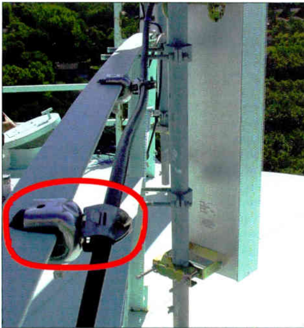
Increased use of beam clamps can reduce or eliminate damage to water tank exterior or interior surfaces or both. Left: A beam clamp secures a coaxial cable. Right: Another type of clamp designed for attachment to structural angles is part of a mounting assembly for two panel-style antennas.
