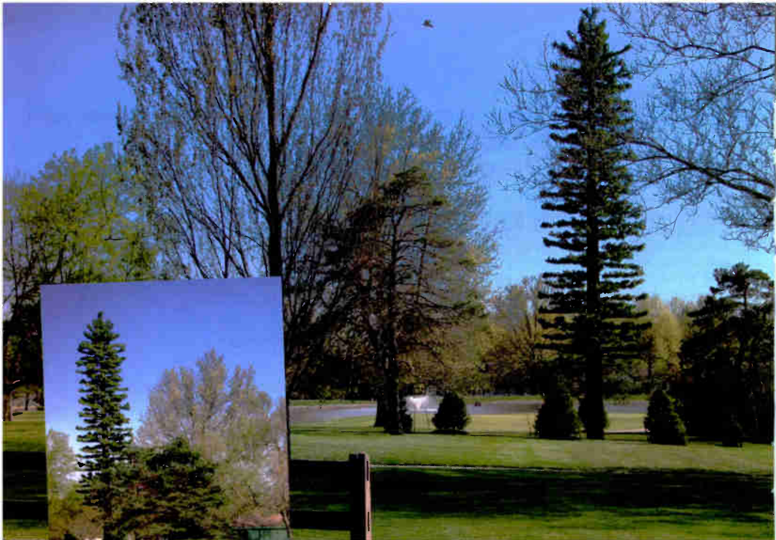
Two views of the monopine concealment pole at the Leawood South Country Club golf course in Leawood, KS. The pre-existing, green-painted maintenance shelter near the base of the pole was lengthened to house base transmitter station equipment. Antenna feedlines between the shelter and the pole are buried. Eight newly planted pine trees circle the pole and are intended to further conceal the site as they grow. Sabre Towers & Poles fabricated the pole.
