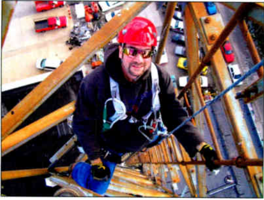
A worker on a tower in Cuddy, Pa., uses fall protection equipment. Photo: Buckingham Manufacturing.
