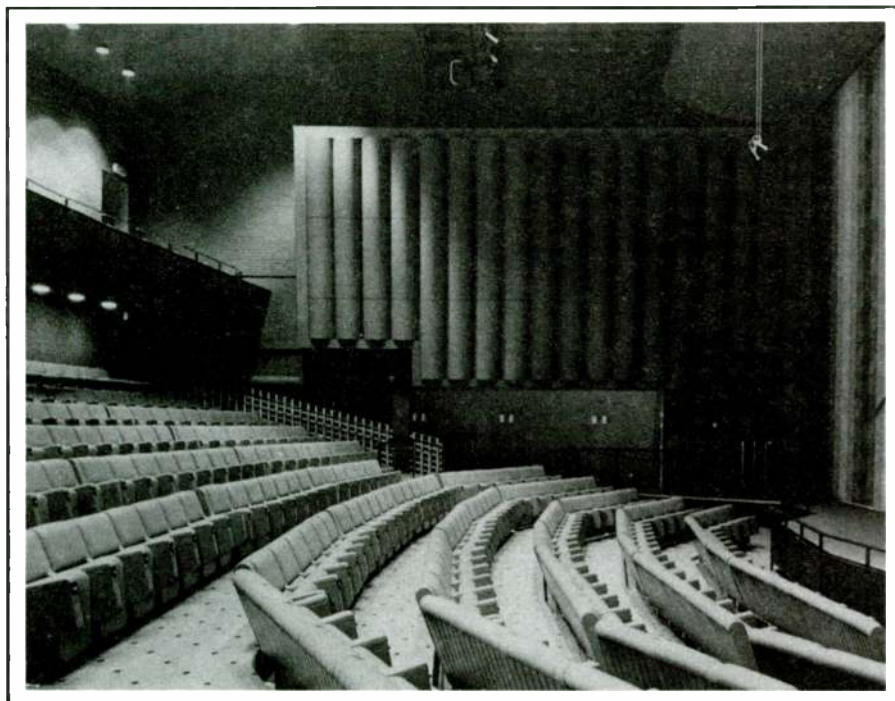
PHOTO 1: The concert hall in Motala, Sweden contains a multi-purpose auditorium with variable acoustics. The cylinders on the side walls are covered by a sound-absorbing material on half their circumferences. With the cylinders so positioned that the absorbent faces the auditorium, the acoustics are suitable for theater performances where voice is the dominant sound. Turning them to present their reflecting sides, to attain a longer reverberation time and more lateral reflections, and enclosing the stage with a concert shell to direct sound into the auditorium, the hall becomes suitable for musical performances.
