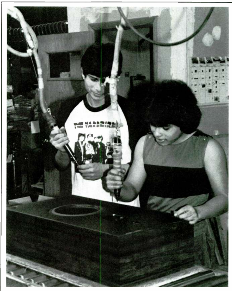
FIGURE 10: The drivers are installed in cabinets on the assembly line.
