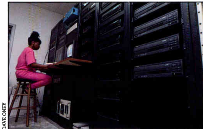
The Rauland-Borg Ranger headend as operated by Betty Wright, Ruffner's media distribution system operator.
