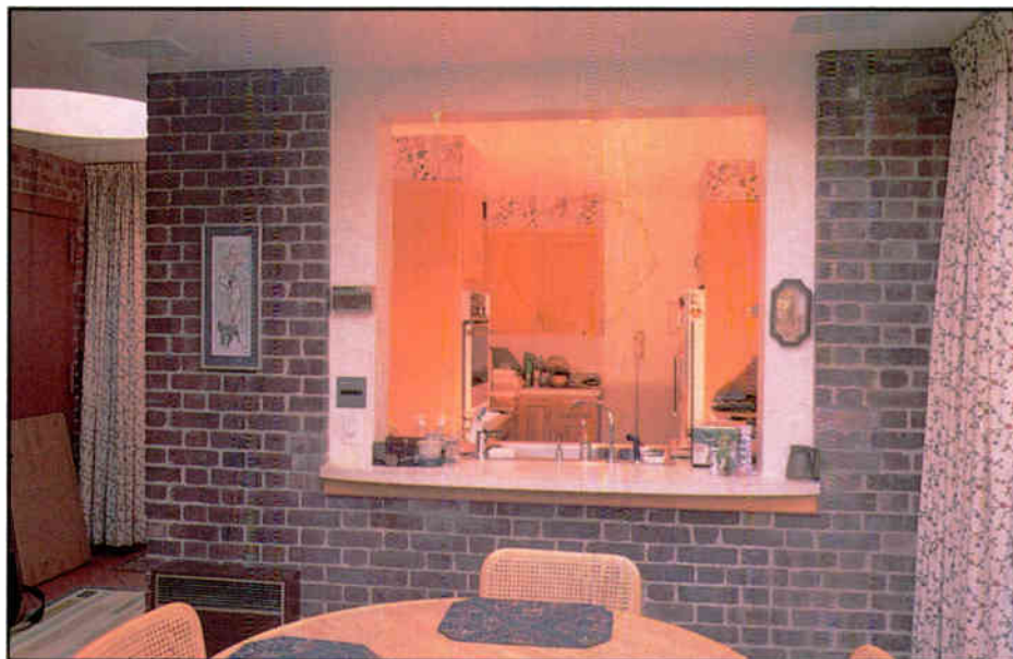
The breakfast eating area with Yamaha in-wall speakers placed in ceiling (upper right) and Yamaha control sensor (left side of pass through).
