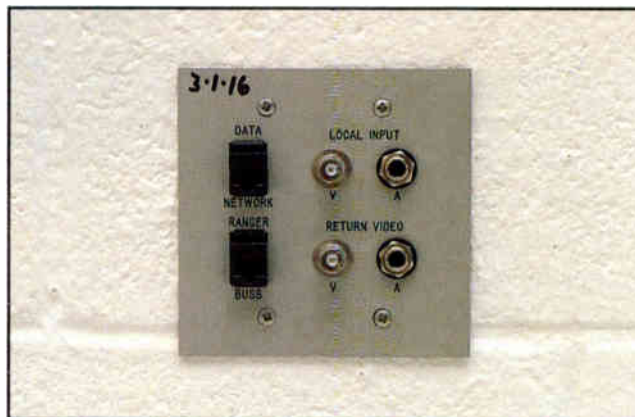
A custom "teacher's panel" for accessing the data network and the Ranger system (fabricated by RCI).
