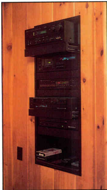
All home theater electronic components are mounted on sliders.
