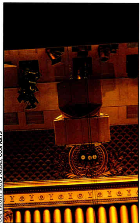
A central cluster, composed of seven Meyer UPA-1B processed sound reinforcement speakers, is suspended over the end of the expanded 40-foot stage used for Pops performances.
