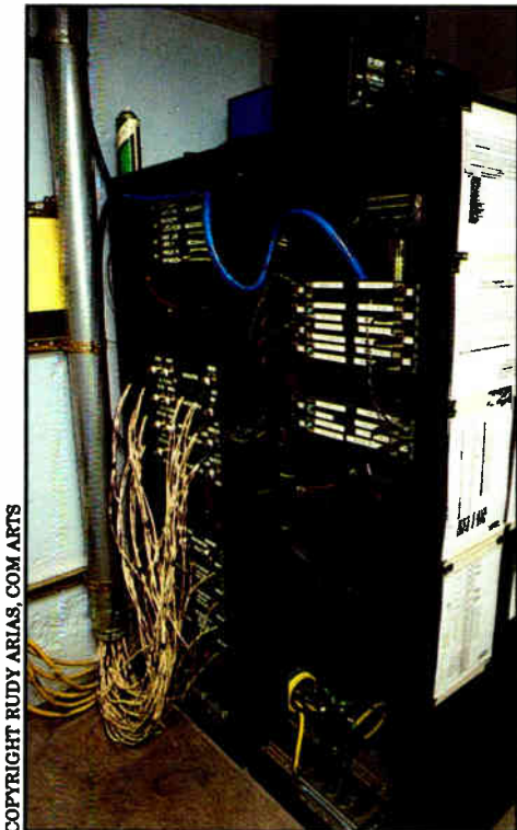
Rear view of the Crown amplifiers showing the wiring involved.
