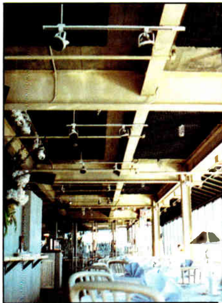
A totally refurbished industrial building, Arthur's Landing has walls of concrete and glass. Sonex I sound-absorbing material was installed to improve acoustics.
