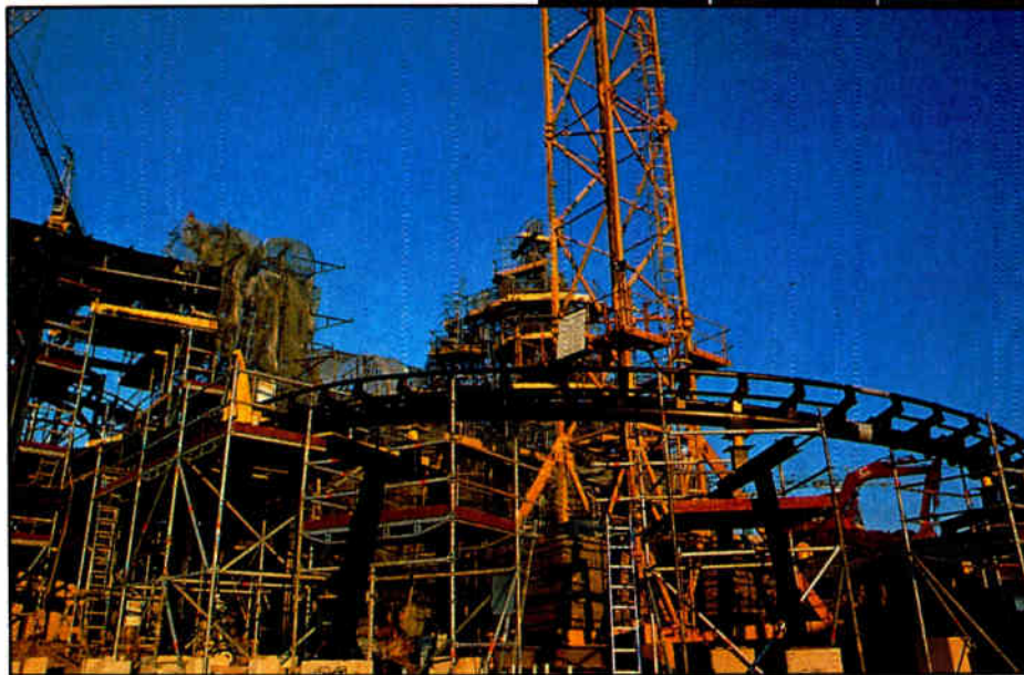
Work in Progress: Big Thunder Mountain.
