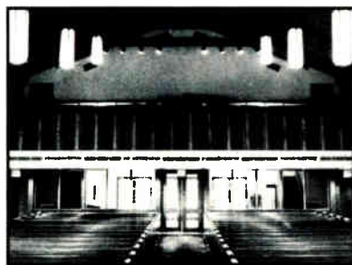
Balcony front after QRD® application
