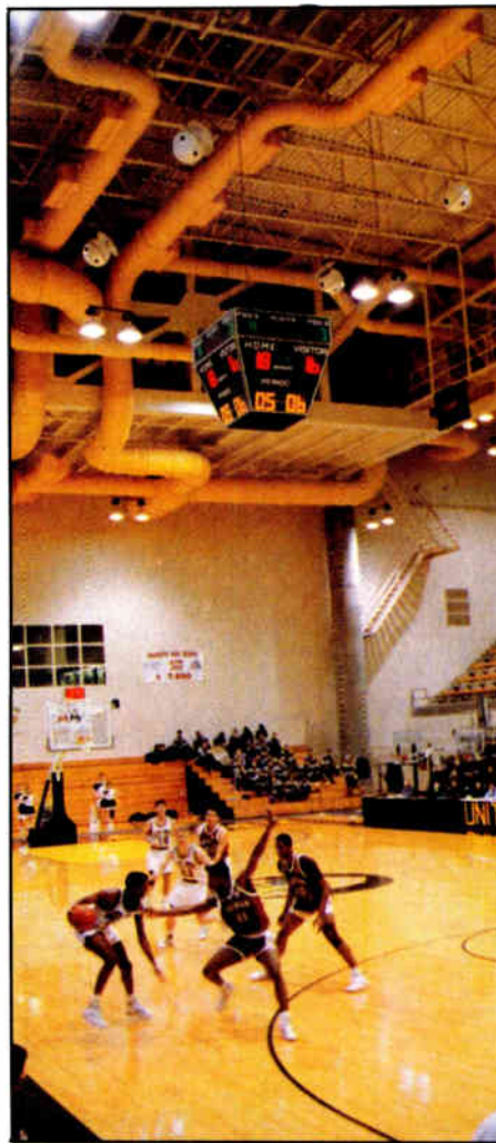
The Holleden Center's basketball arena.
