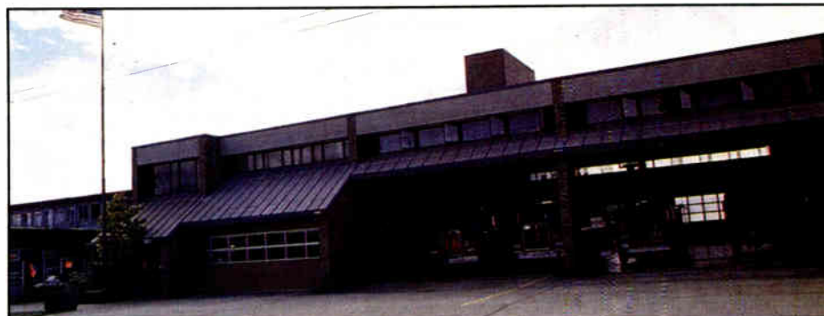
The Seattle Fire Department has recently completed a major upgrade.
