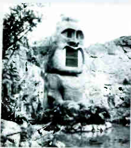
(Top) During the actual installation of the various components in the tiki. (Bottom) The completed Menehune Tiki speaker system.
