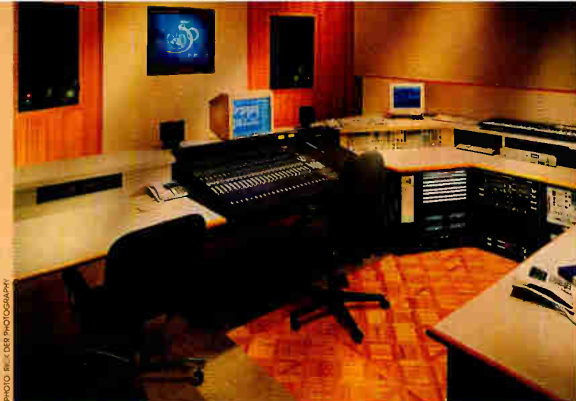
As part of a complete facility overhaul, San Francisco's Robert Berke Sound remodeled its Studio B, working in consultation with original designer Randy Sparks of RLS. Completed in June '95, the post room now includes an automated Otari Status console, a 24-track Timeline DAW, 80, 16 tracks of Tascam DA-88 and JBL surround monitoring.
