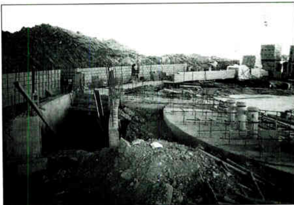
Concord Pavilion FOH position during construction
