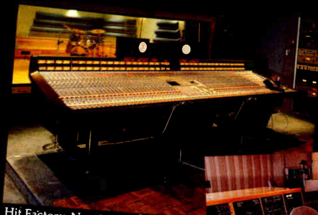
Hit Factory, New York (4 SSL rooms)
