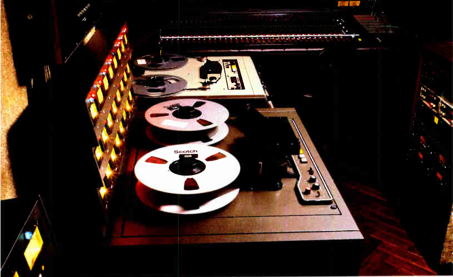
System shown: Sony JH-24 multitracks, JH-110C recorder/reproducer, JH-636 AF/LM console, PVM 1910 monitor. Facility: Reelsound Mobile Recording Unit, Austin, TX.
