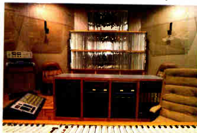
Rear wall showing diffusion-reflection
