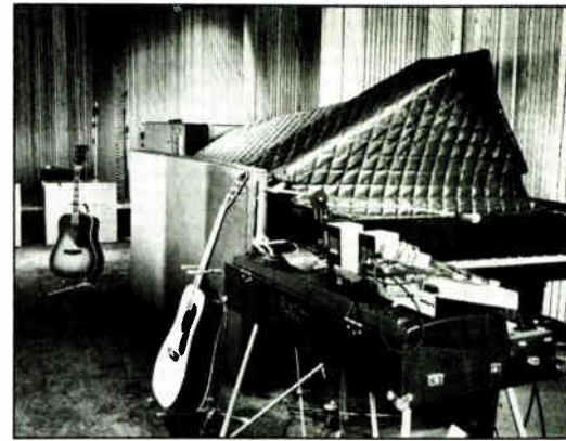
Irregularly shaped wall cavities of slot absorber/diffusers and bass traps
