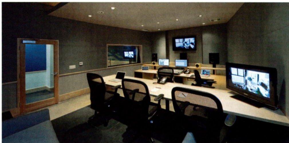
740 Sound Design (L.A.) was designed by Peter Grueneisen (above) of studio bau:ton and nonzeroarchitecture, and features an Avid CL24 and a Genelec 5.1 surround sound system. Studio photo courtesy: Juergen Nogai.
